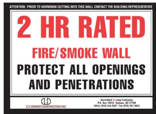
Example of a label for fire / smoke resistance rated assembly
